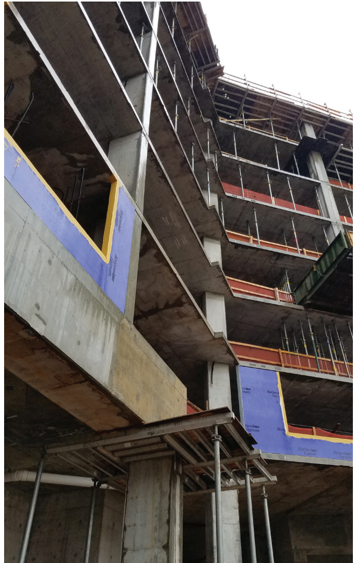
Fig. 8—Transfer girder picking up column at second floor.
