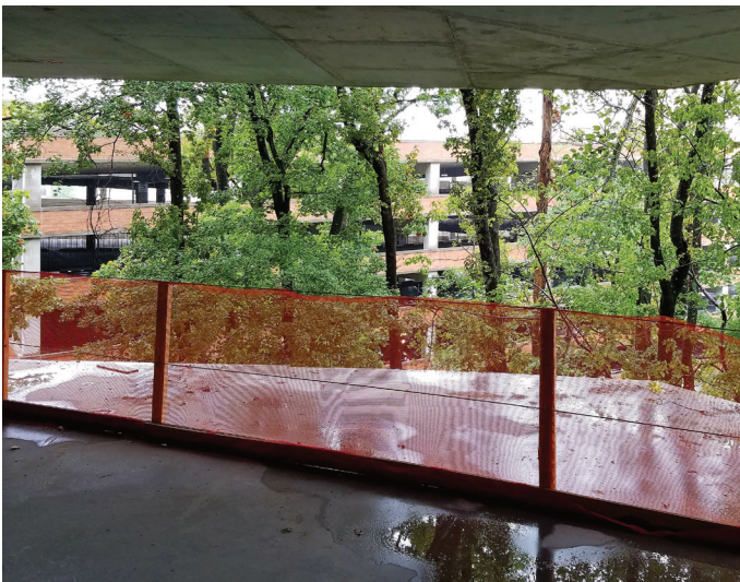
Fig. 7—Twelve foot (3.7 m) long cantilever balconies at building corners.
