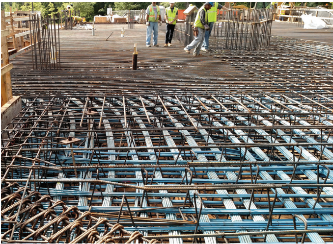
Fig. 6—Transfer mat ready to place.
