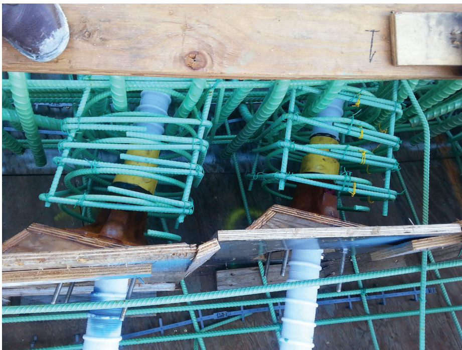
Fig. 6—Stress end anchorages and formwork.
