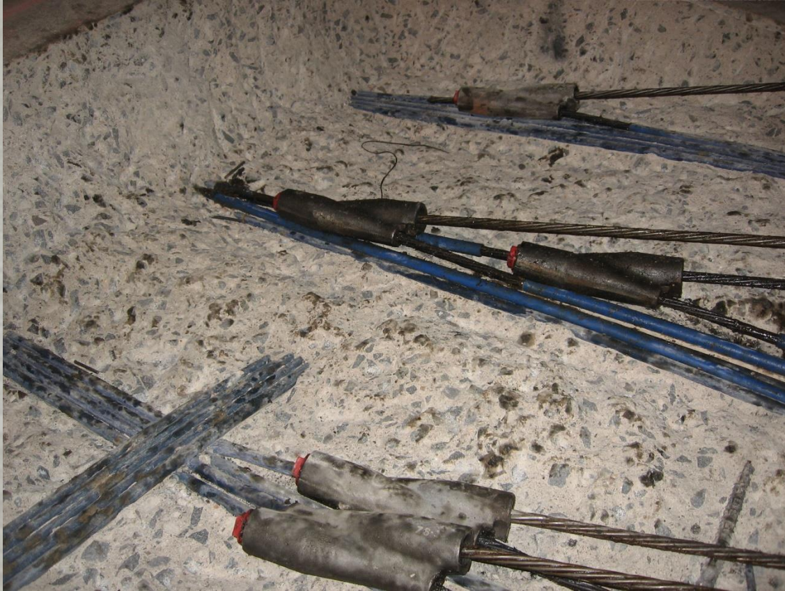
Center Stressing Anchor (Lok Coupler)
