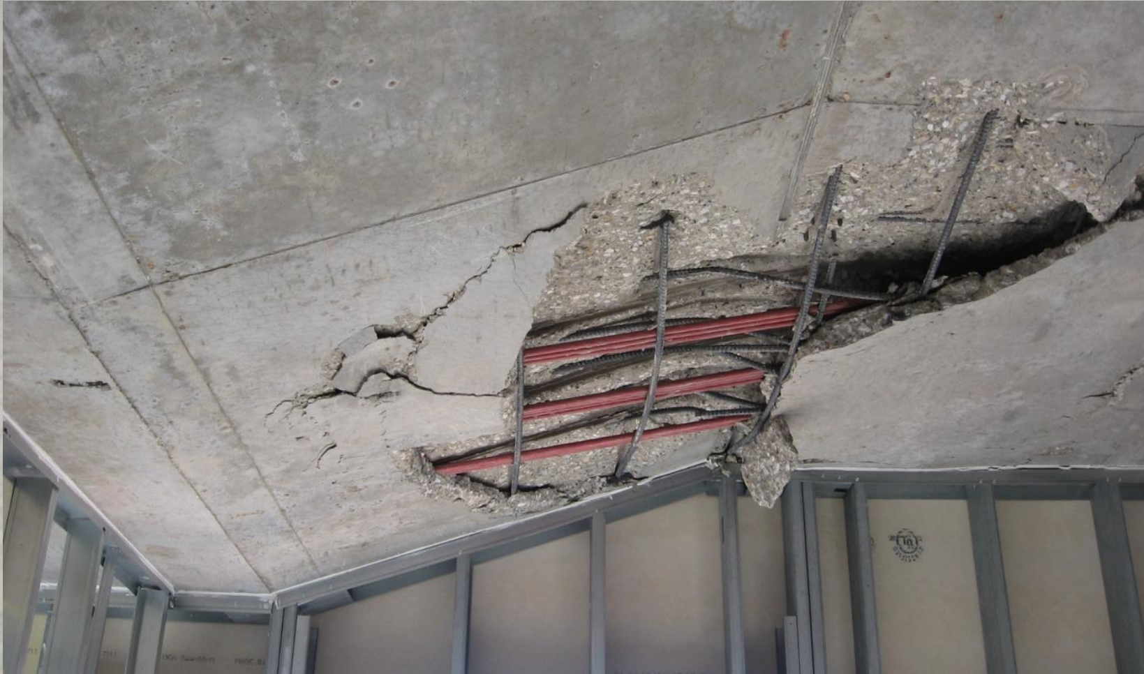
Blowout at slab fold
